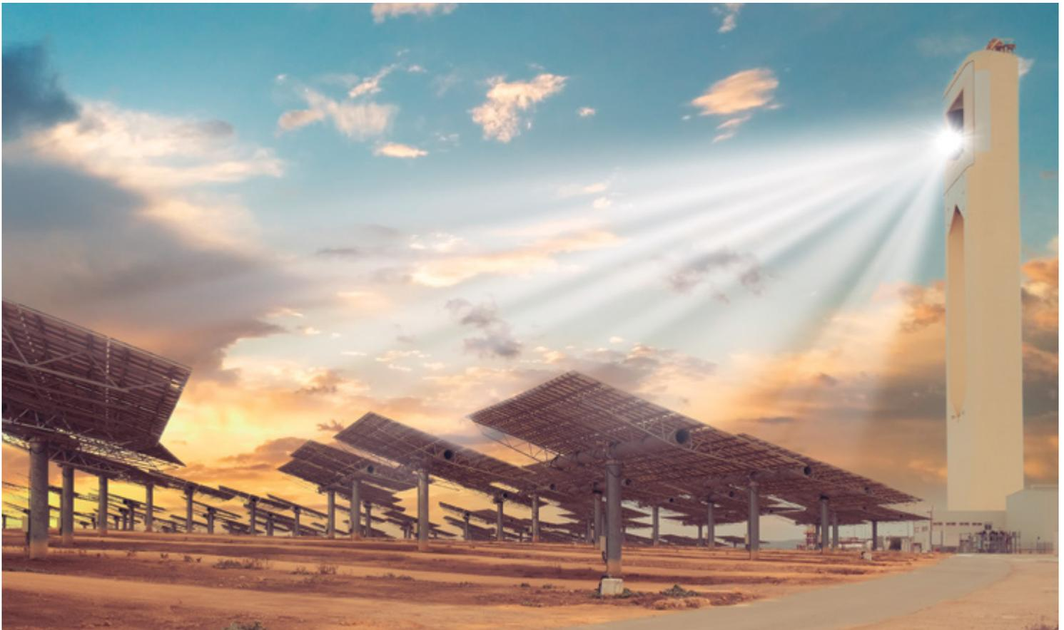
Gemasolar Concentrated solar power plant CSP, system generate solar power using mirrors lenses to concentrate large area of sunlight onto receiver. Seville, Andalusia.
